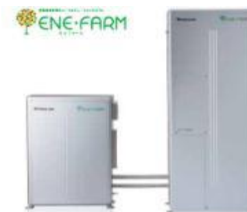
Residential polymer electrolyte fuel cell (PEFC) cogeneration system
